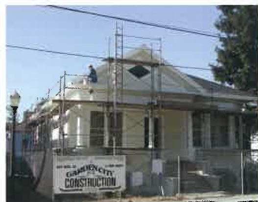
Pasetta House under renovation, fall 2004.
