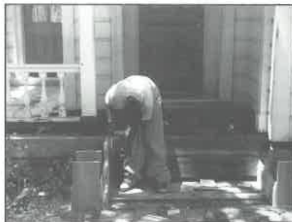
HSJ staff person repairs the steps of the Chiechi House.
